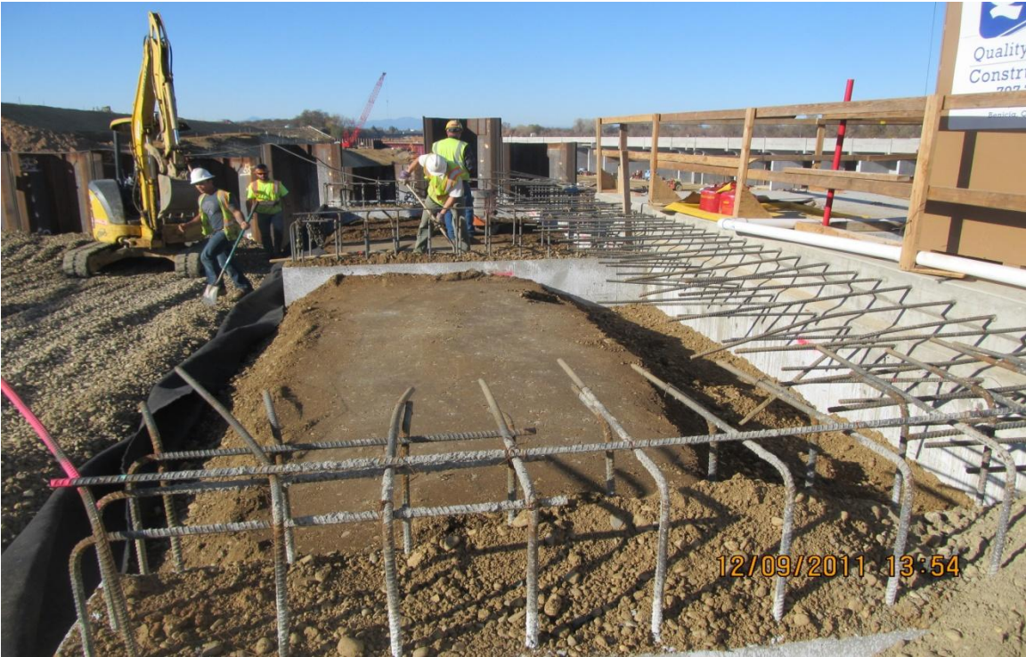
Balfour Beatty subcontractor Meyers backfilling at the Pumping Plant.
