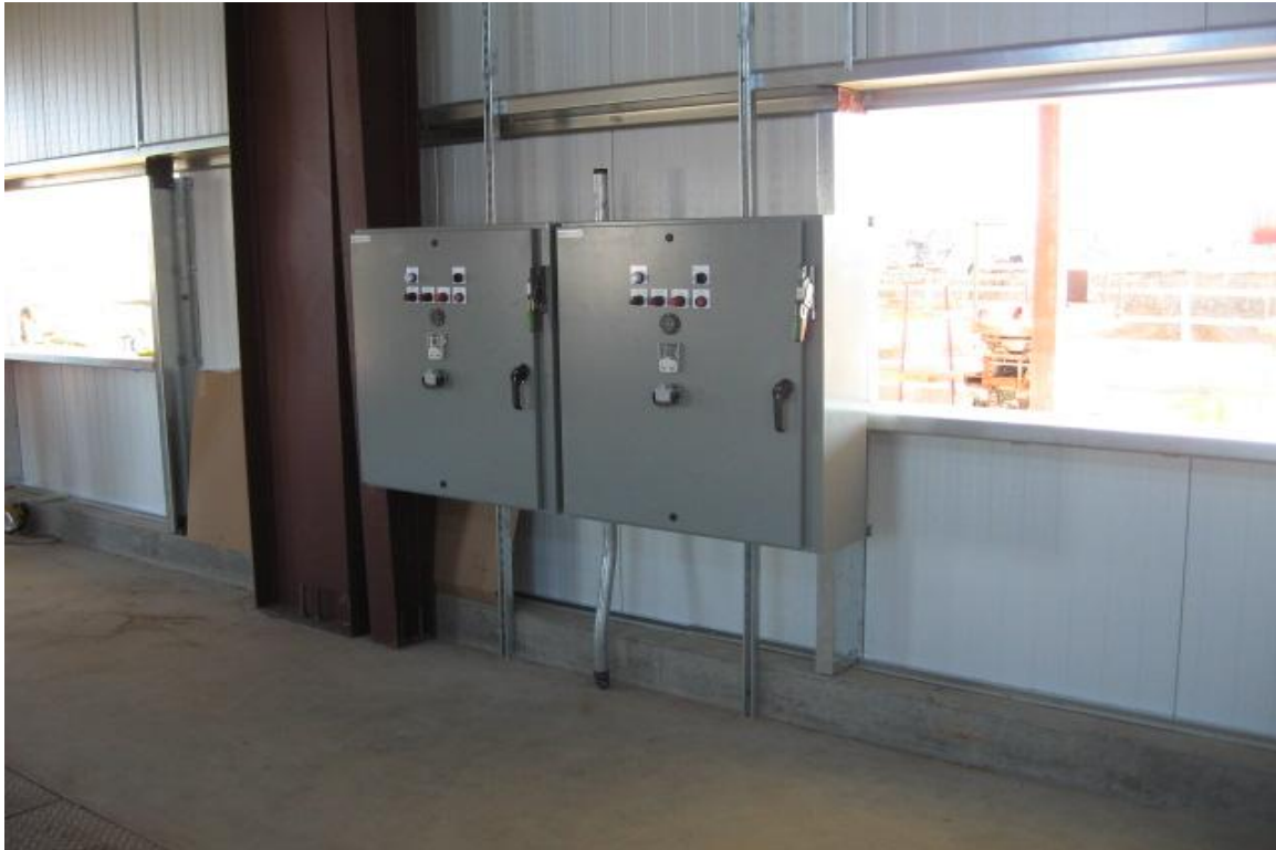
Balfour Beatty subcontractor Central Sierra Electric installed Fish Screen control panels.
