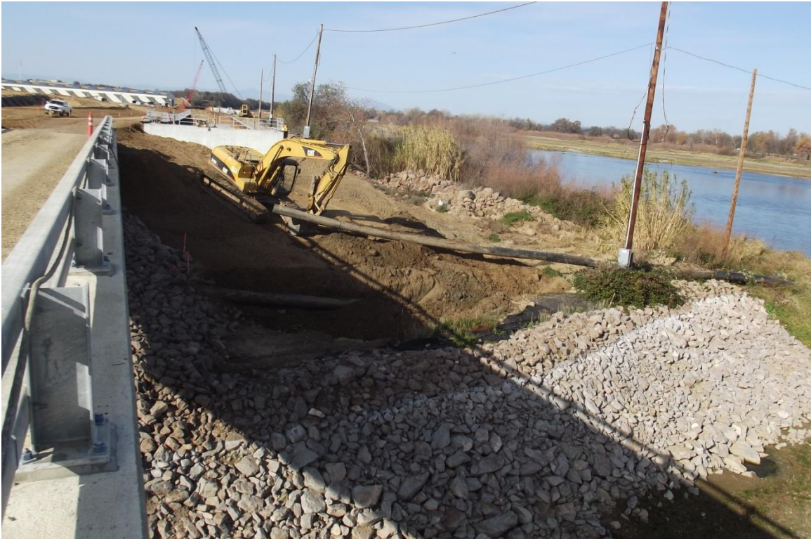
West Bay Builders subcontractor Meyers removing temporary pipeline.
